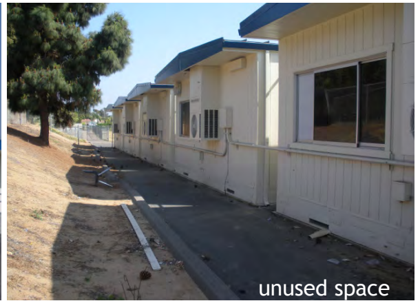
existing modular classrooms at palmquist elementary
